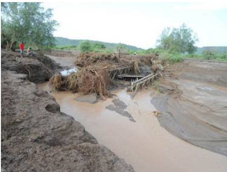
The bridge at Lokurwa
