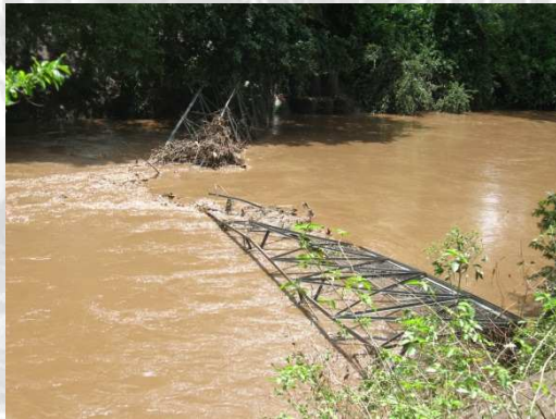
The Kuron Pedestrian Bridge in the water
